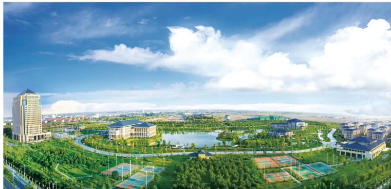
特变电工总部科技研发基地（新疆昌吉） TBEA Headquarter Scientific and Technological R&D Base (Changji City, Xinjiang)
