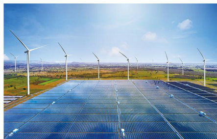
▲ 上海光伏太阳能电站 Shanghai Photovoltaic Solar Power Station
